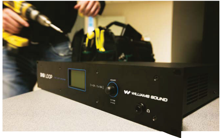
Installing the Digi-Loop 210
